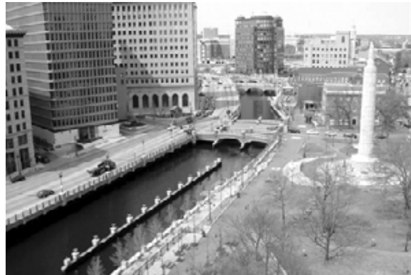
River after roadway with new bridges and relocated World War I Memorial
