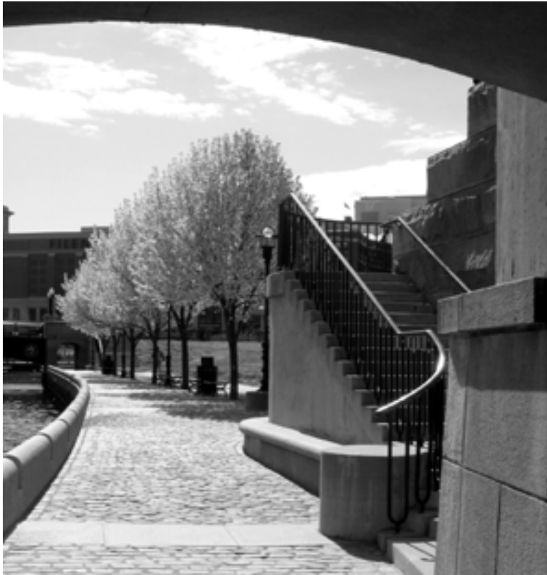
Walkway with stair from street
