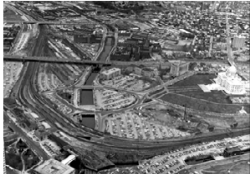
Aerial with railroad and roads before relocation
