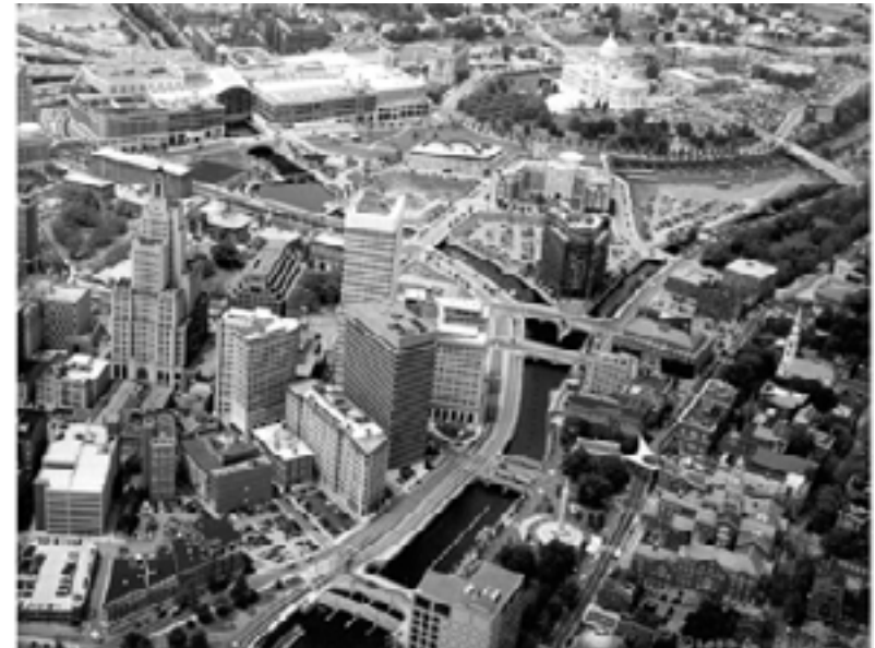
Completed Providence River relocation
