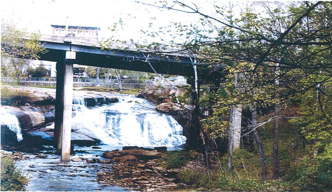
Camperdown Vehicular Bridge 1960 - 2002
