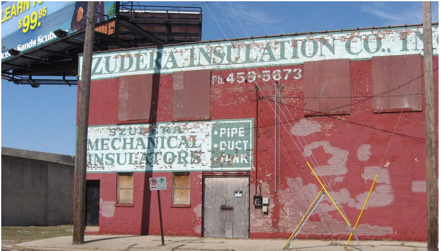
Previous Building South Side
