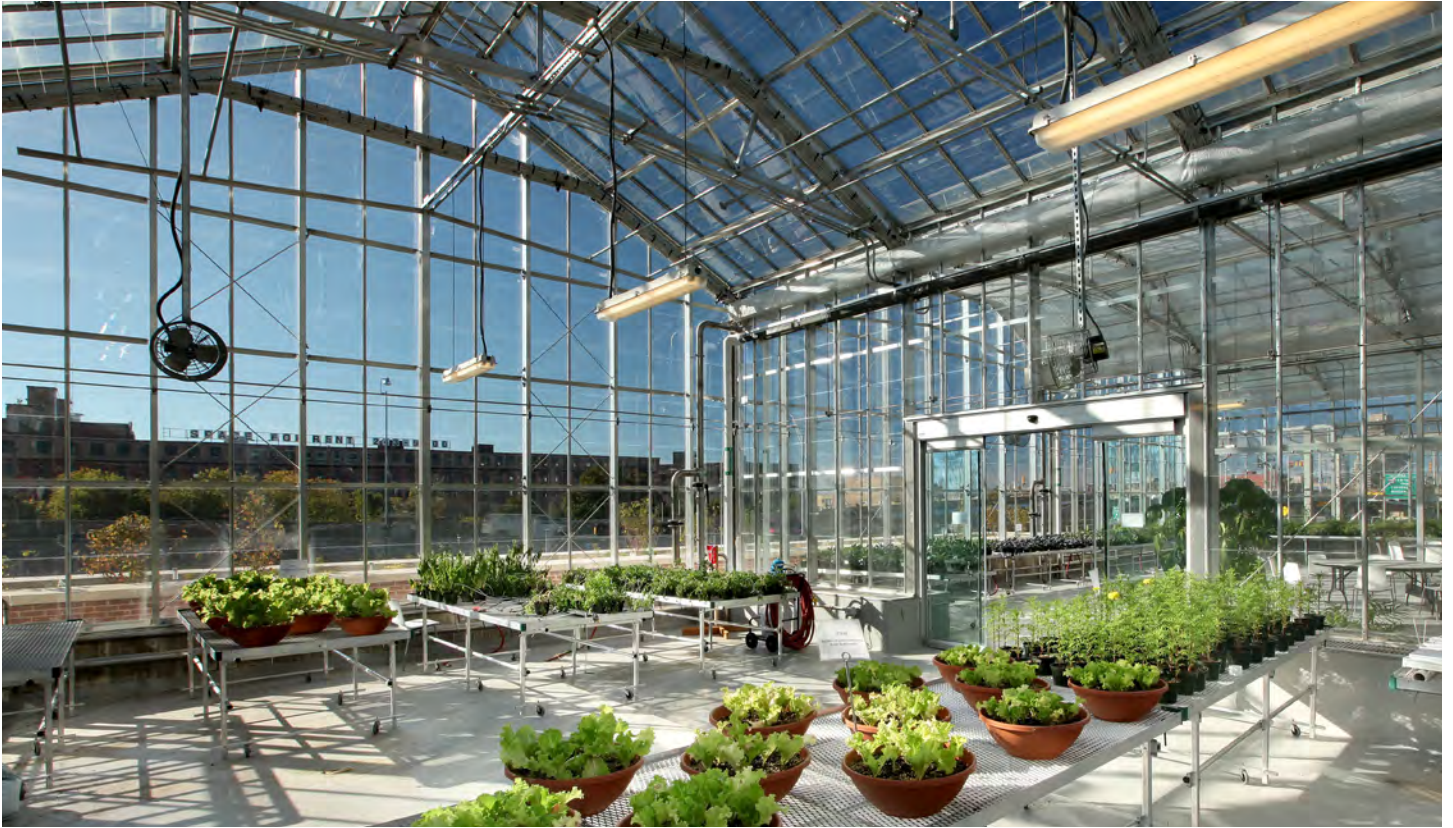
The Downtown Market features two independently controlled greenhouses using the Priva Integrated Process Management System.
