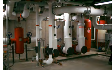
Geo-thermal well system.
