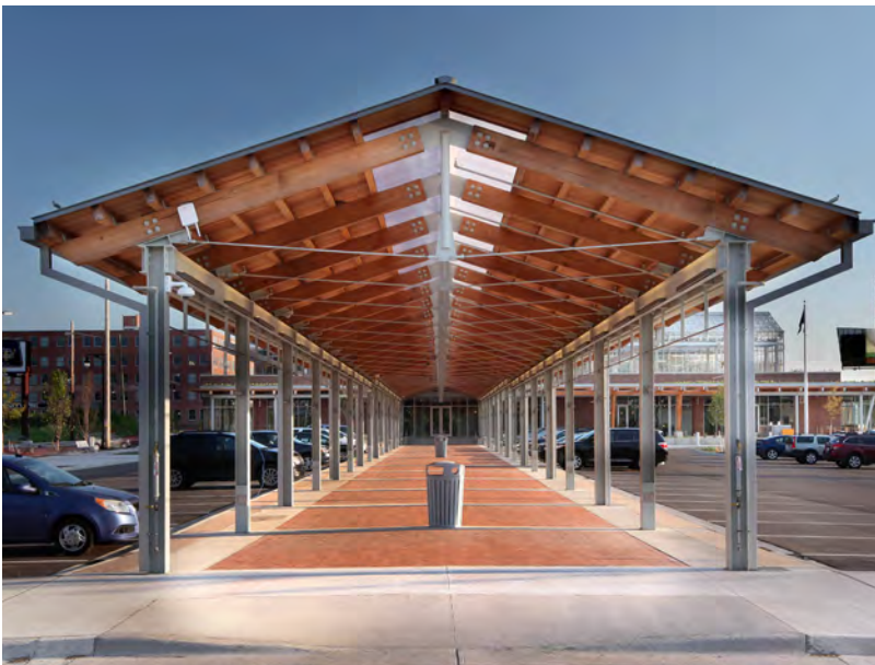
Market Shed features snowmelt, skylights, and recycled wood from previous buildings.
