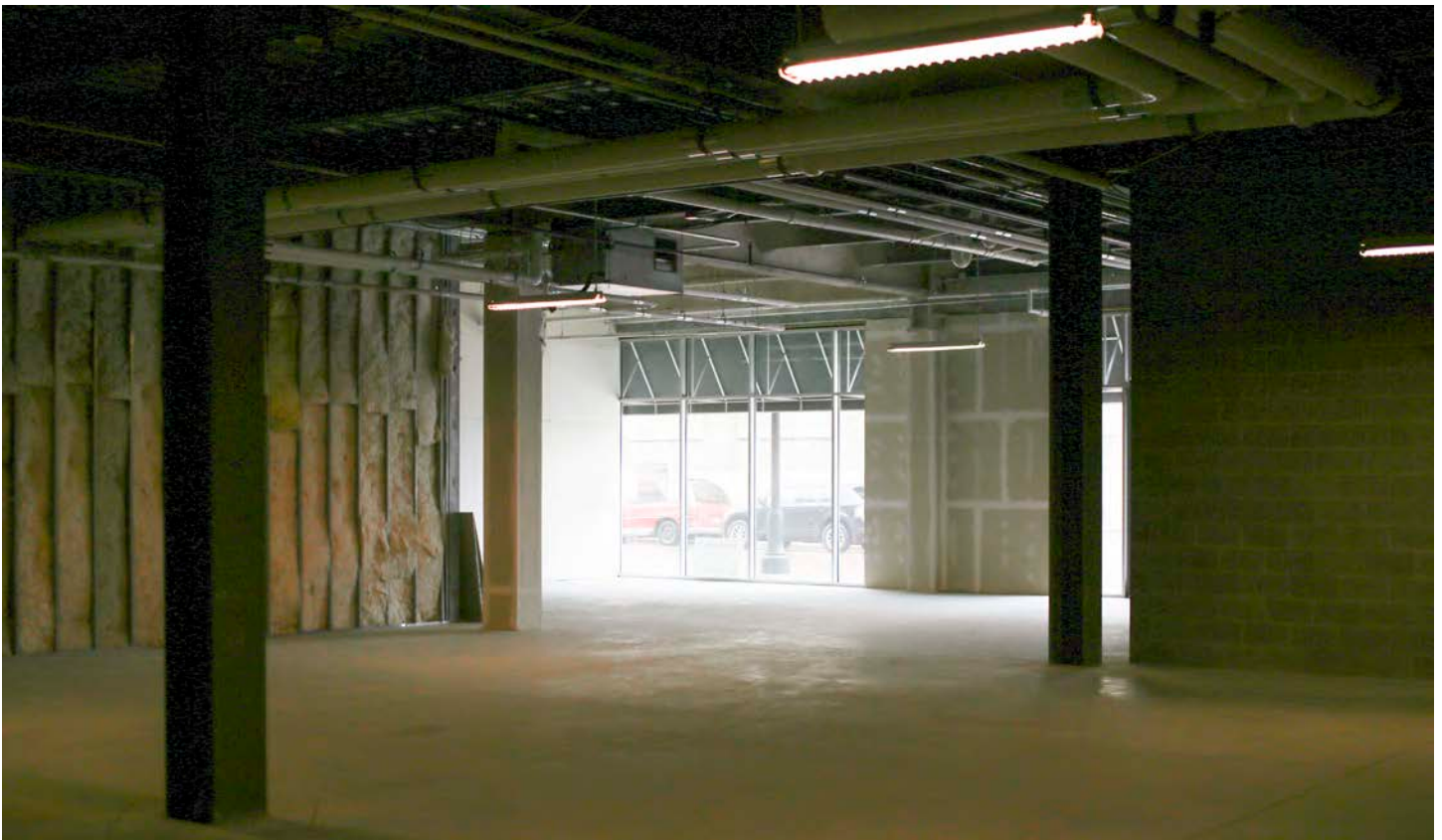
The first floor remaining commercial space is just under 5,000 square feet and is adjacent to the Market's loading dock.
