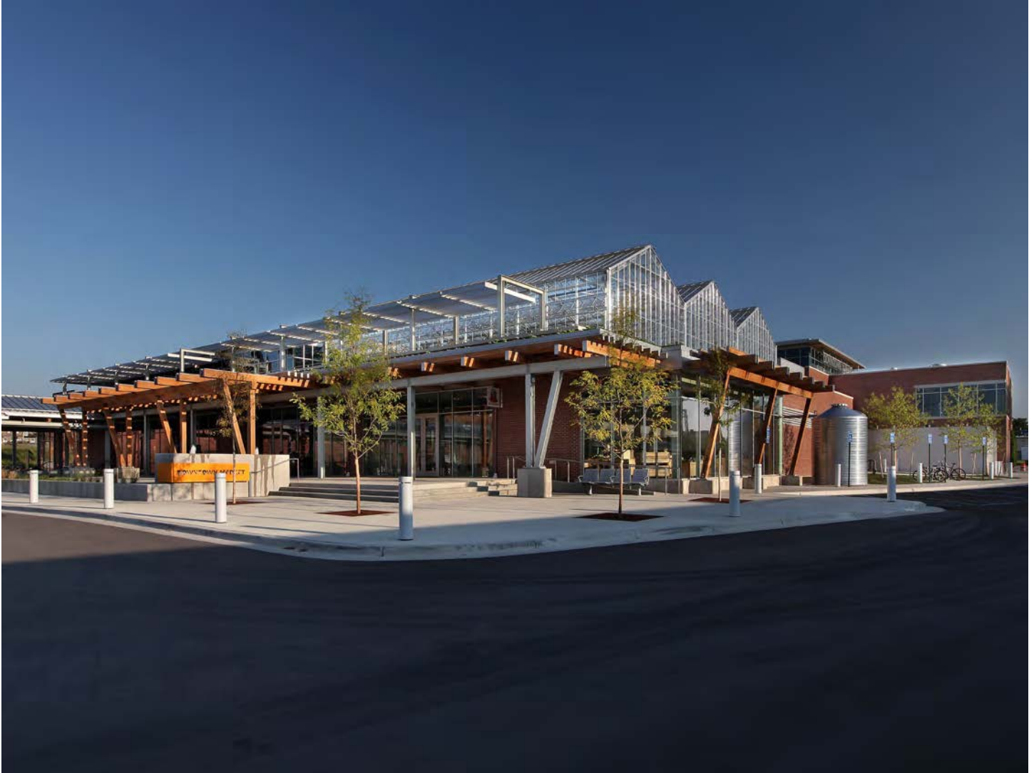
Exterior of Market, concrete foundations from previous buildings ground up and used as parking lot base.
