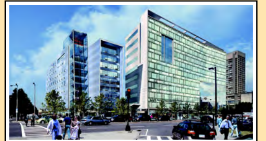
Crosstown Development New construction of mixed-use development.
