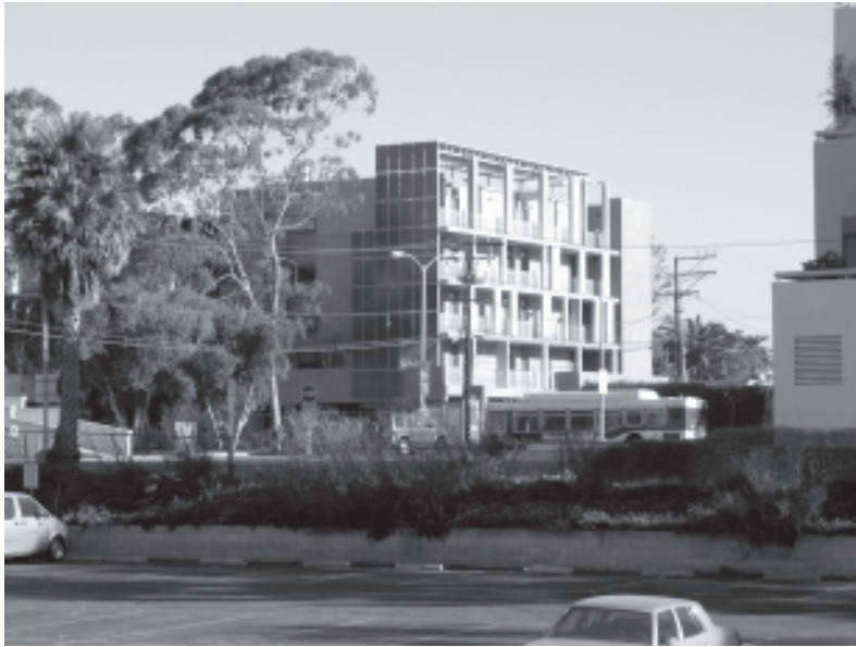
Colorado Court south elevation
